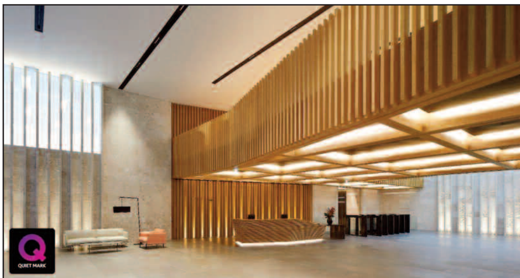
The BASWA Phon acoustic plaster system is both Quiet Mark certified and listed on NBS. © Hufton + Crow.
