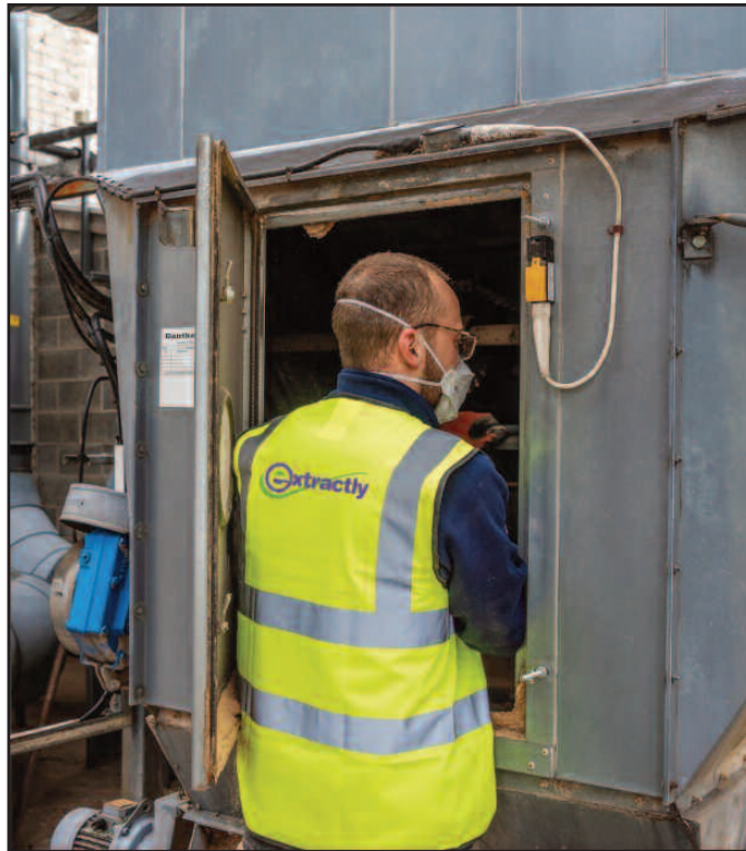
Internal inspection of customer's filter unit.
