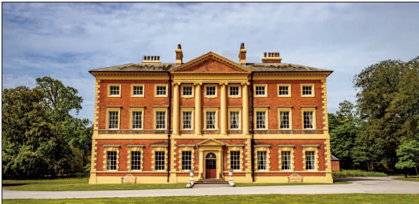
Above, East elevation, Lytham Hall. Below, Jacobean bedroom, Lytham Hall.
