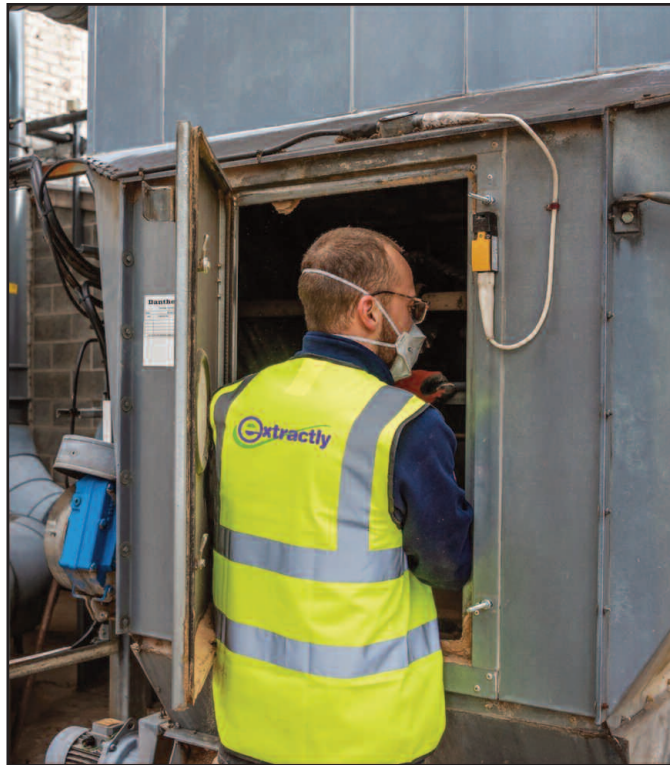
Internal inspection of customer's filter unit.
