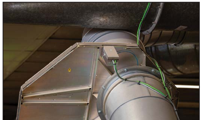
Ecogate® automatic motorised damper retro-fitted into 400 mm diameter ductwork.
