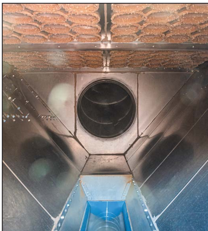
Internal view of the filter unit in operation shows dust and woodwaste collecting on the tubular filter bags and rotary valve located at the bottom of the hopper.
