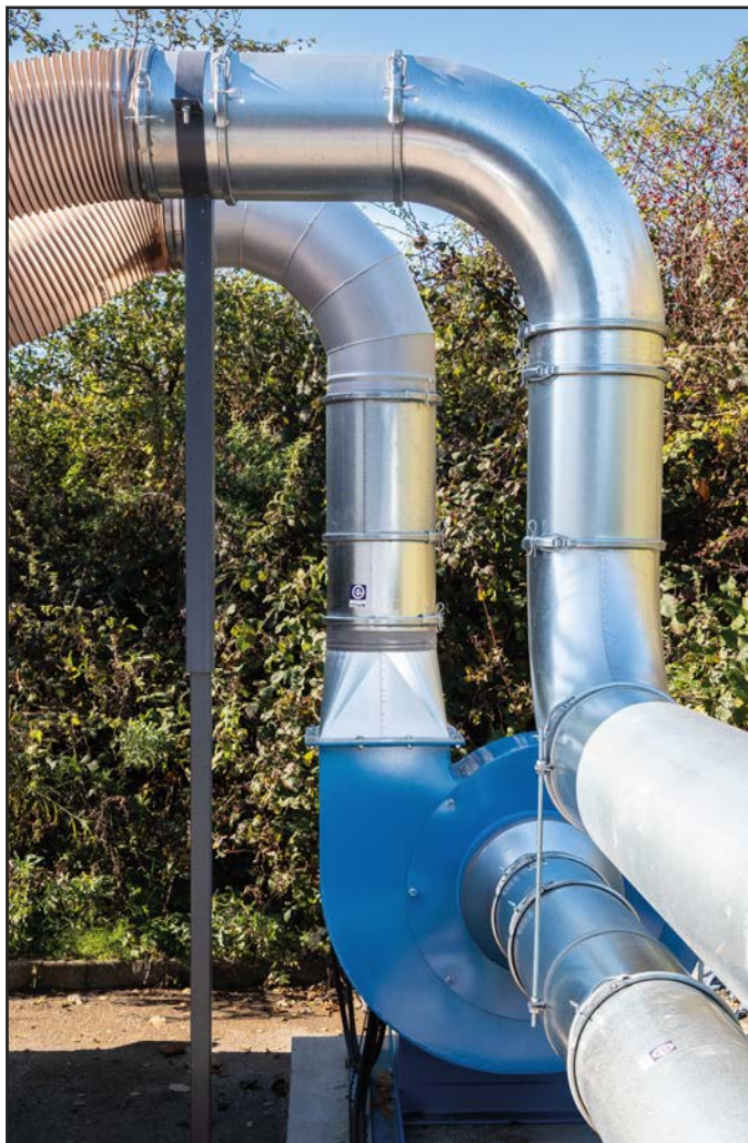
15 kW transport fan blows waste into storage container.
