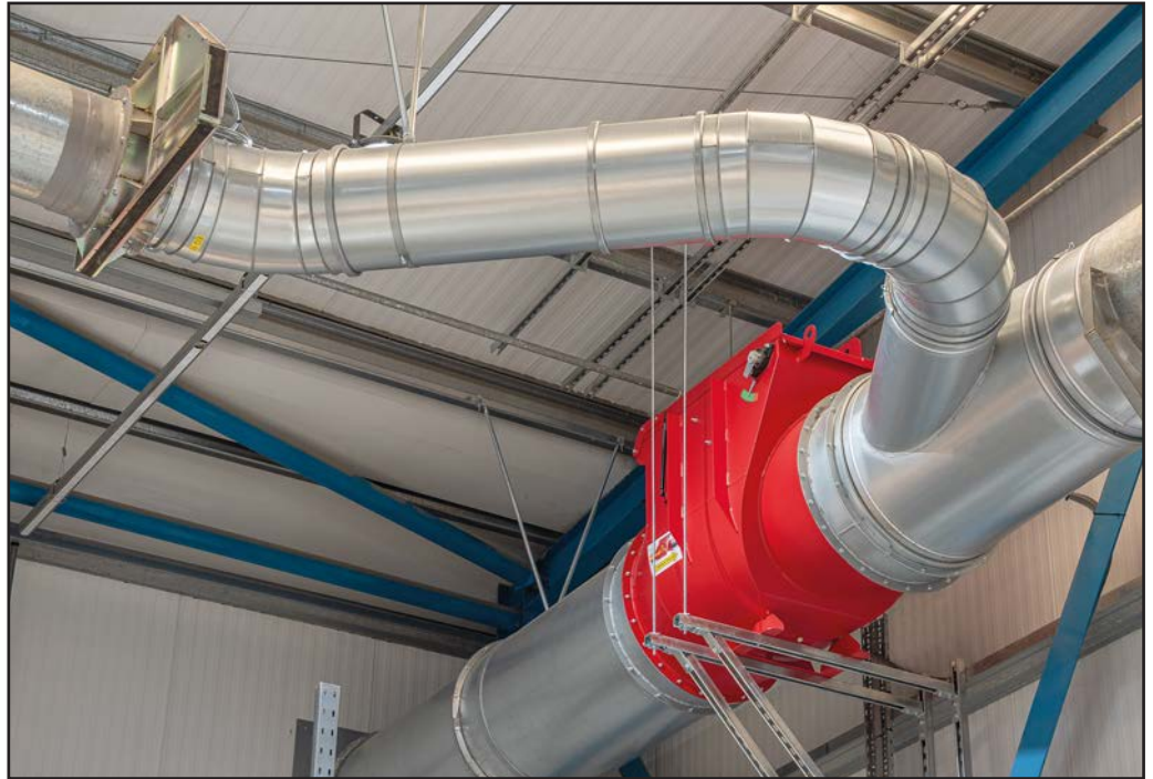
ATEX isolation valve prevents pressure wave and flames travelling into the factory.
