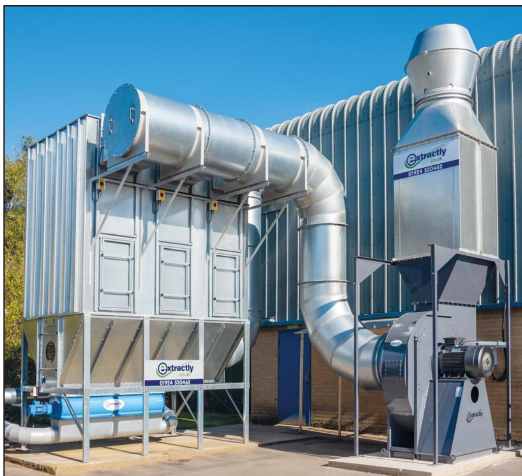
33,000 m 3 /hr capacity ATEX filter unit with main fan fitted to 'clean side' of the filter unit for maximum efficiency. Noise is attenuated by the silencer fitted above the fan.
