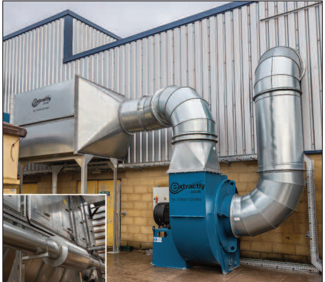
Bespoke absorptive silencers significantly reduce noise levels from the 90 kW main fan.
