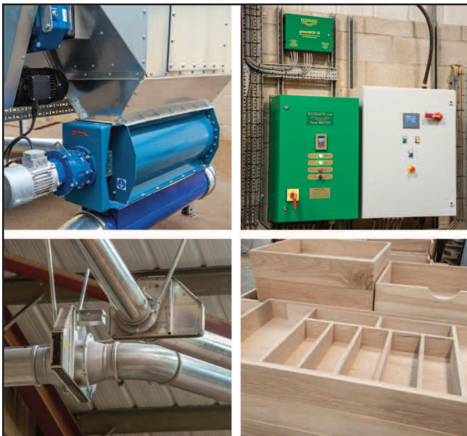
Top left: Rotary valve unit discharges filtered waste pressure-free.
