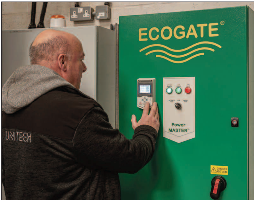
The Ecogate PowerMASTER, specifically designed to optimise an Ecogate-controlled extraction system, features an easy-to-use keypad with high contrast screen for easy configuration, and can automatically manage fan start-up and shutdown.
