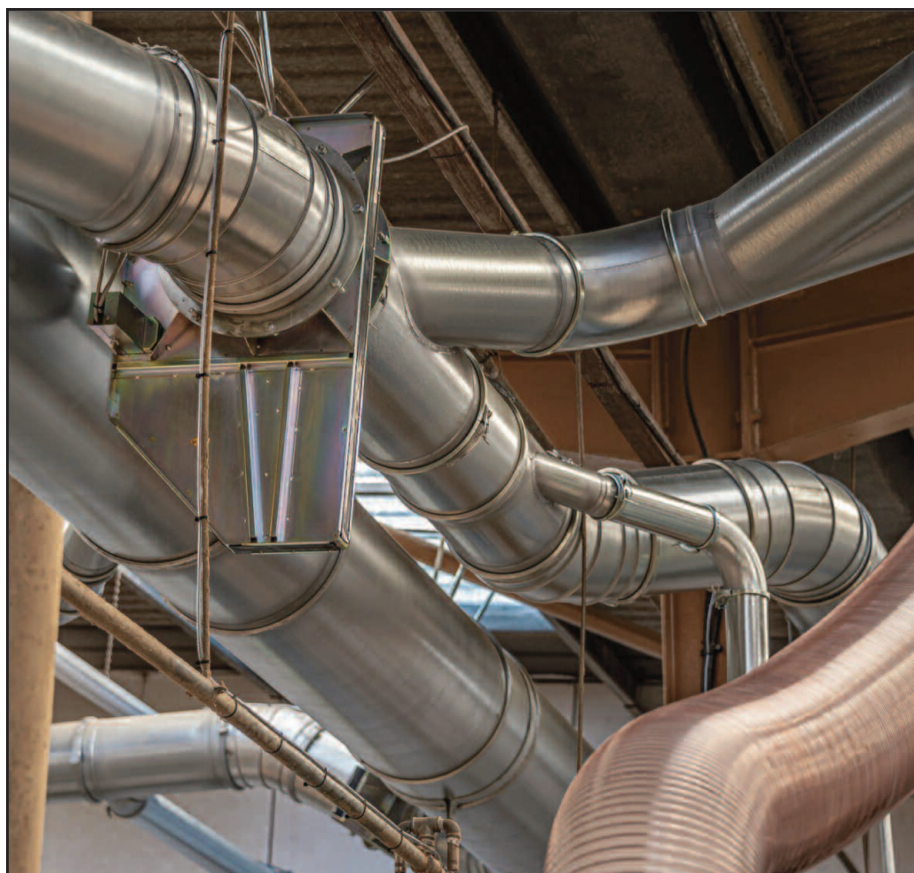
Ecogate's motorised dampers integrated into the Nordfab QF ductwork system automatically open and close as machines come on or offline.
