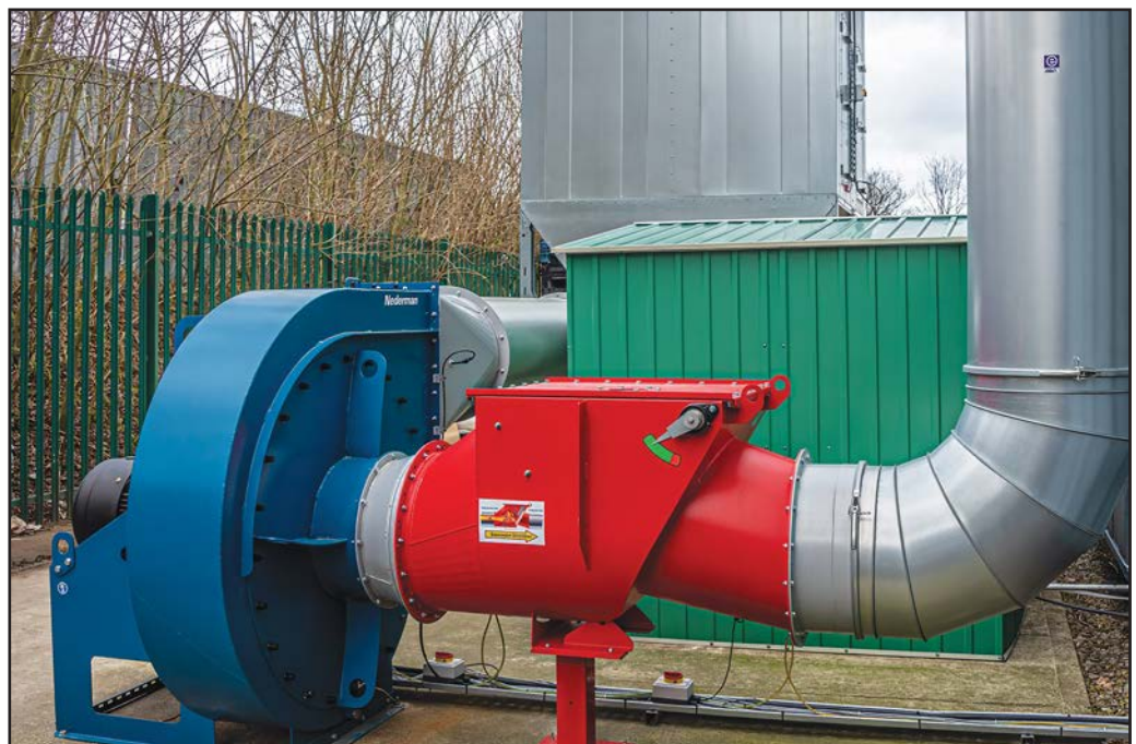
30 kW main fan draws dust-laden air from the high-speed machinery, through the Nordfab QF ductwork system, via the non-return explosion isolation valve, and into the filter unit.
