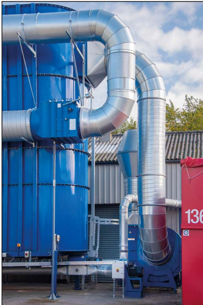
Newly-commissioned, the pre-owned filter and fan unit are in 'as new' condition.
