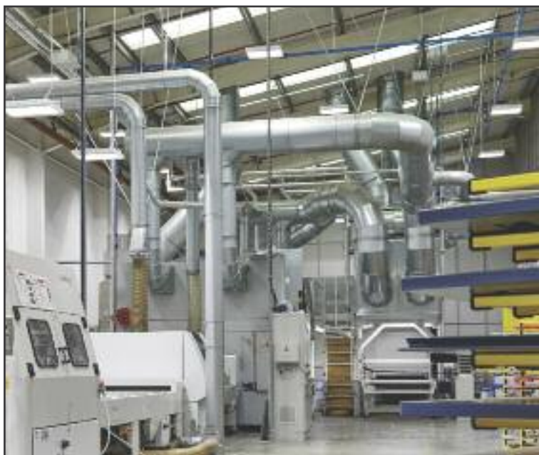
Extraction ductwork installed in Omega's paint shop. / Photo: Omega PLC
