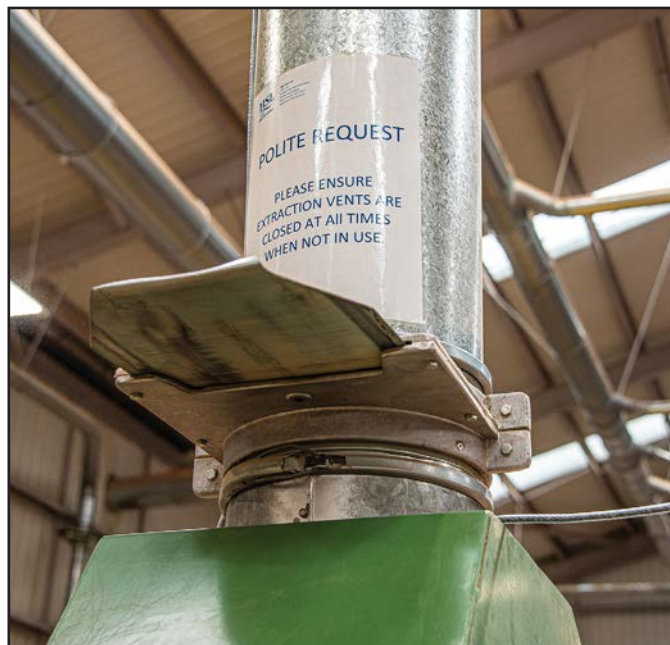
"Polite Request" notice is no longer needed at HSL — the old manual gates are now left permanently open as Ecogate dampers do the job automatically.
