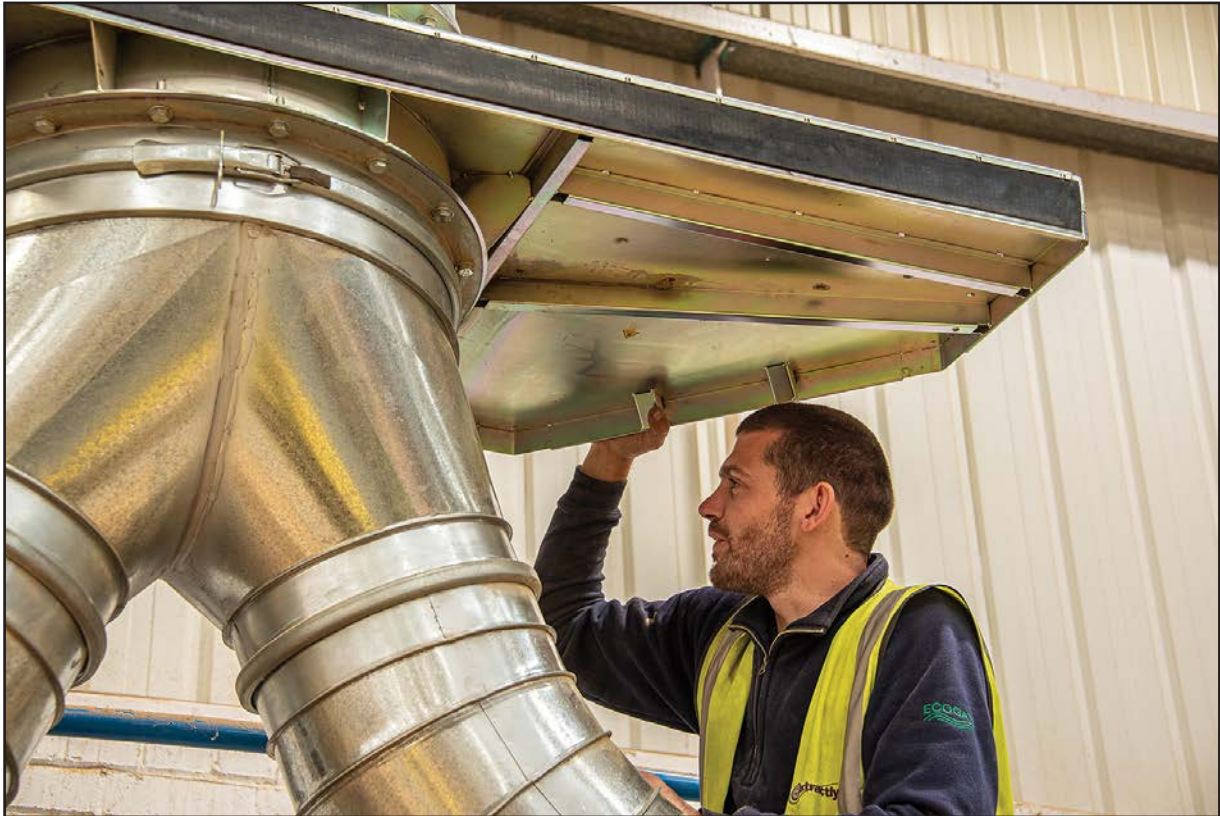
Final checks on a 560 mm diameter automatic Ecogate damper fitted to a 'vintage' Rye Rotary Shaper.
