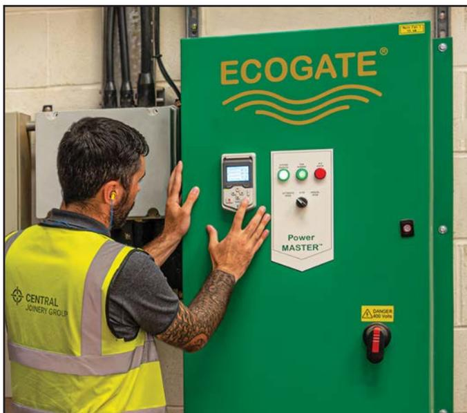
*As instructed by the greenBOX® NXT controller, Ecogate® Power MASTER Variable Speed Drive units adjust fan speed to exactly match extraction demand on each of the 3 lines.*
