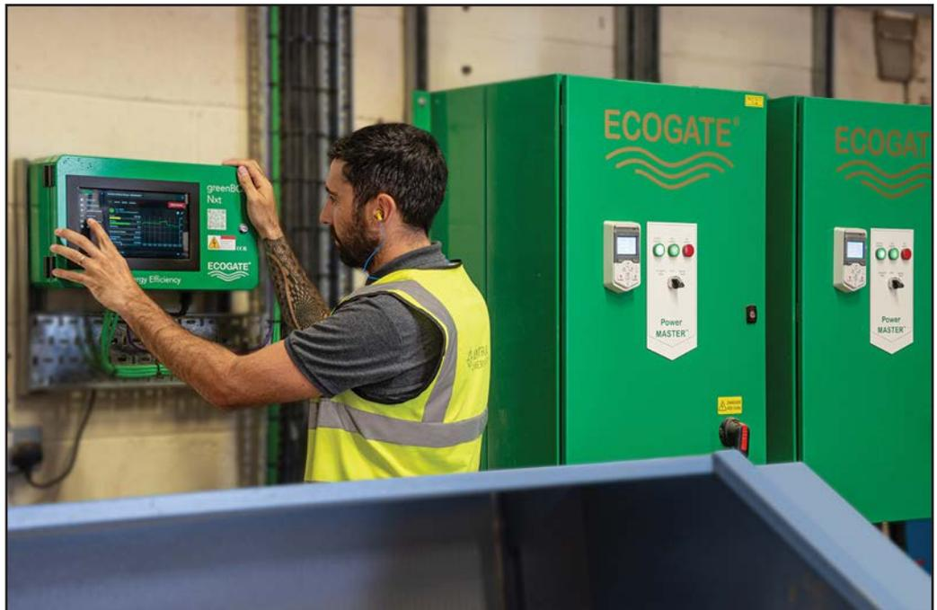
*Operations director Kyle Archbold interrogating real-time system performance data on the highly intelligent Ecogate greenBOX® NXT controller which has the capacity to monitor and control an extraction system with multiple main fans and up to 72 individual workstations.*
