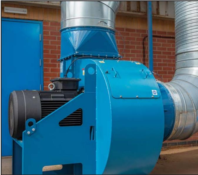
**Extractly supplied and installed a new 55kW Nederman main fan at Central Joinery Group's head office at Swadlincote.**
