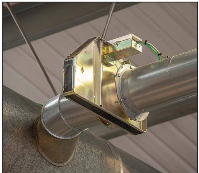
*Extractly Ltd retro-fitted over 20 Ecogate® motorised dampers into the existing ductwork system at Central Joinery.*
