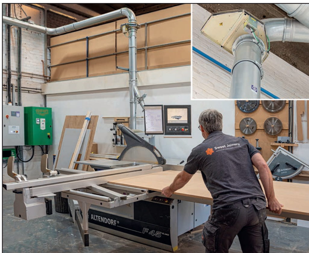
Above: Ecogate® motorised dampers open and close automatically as machines come on or off-line.
