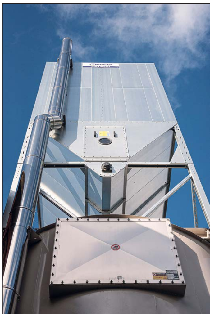
Above: Ecogate® motorised dampers open and close automatically as machines come on or off-line.
